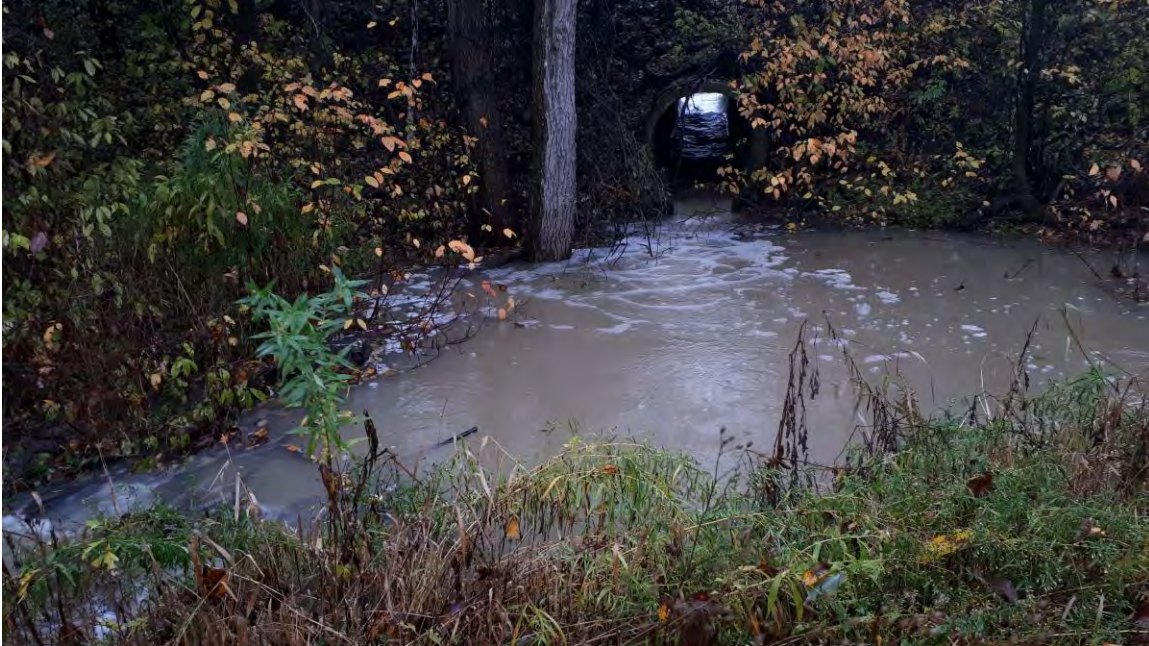
Figure 2. Perched culvert outlet at upstream extent of subject property (facing east).
