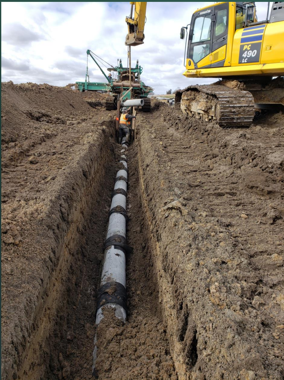
Tile Installation by means of Wheel Machine
