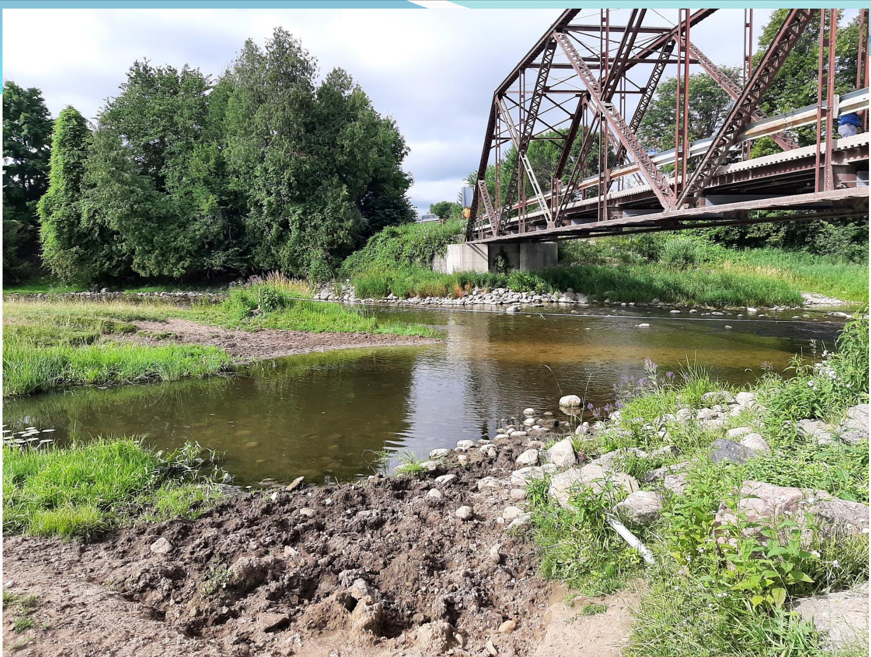
Photo of new alignment looking south from north side
