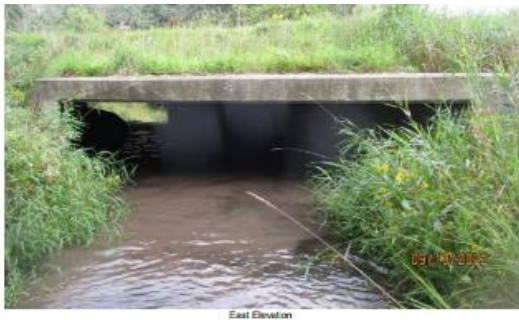
Figure 29 M080 Clyde Line Culvert (BCI=53 Fair)
