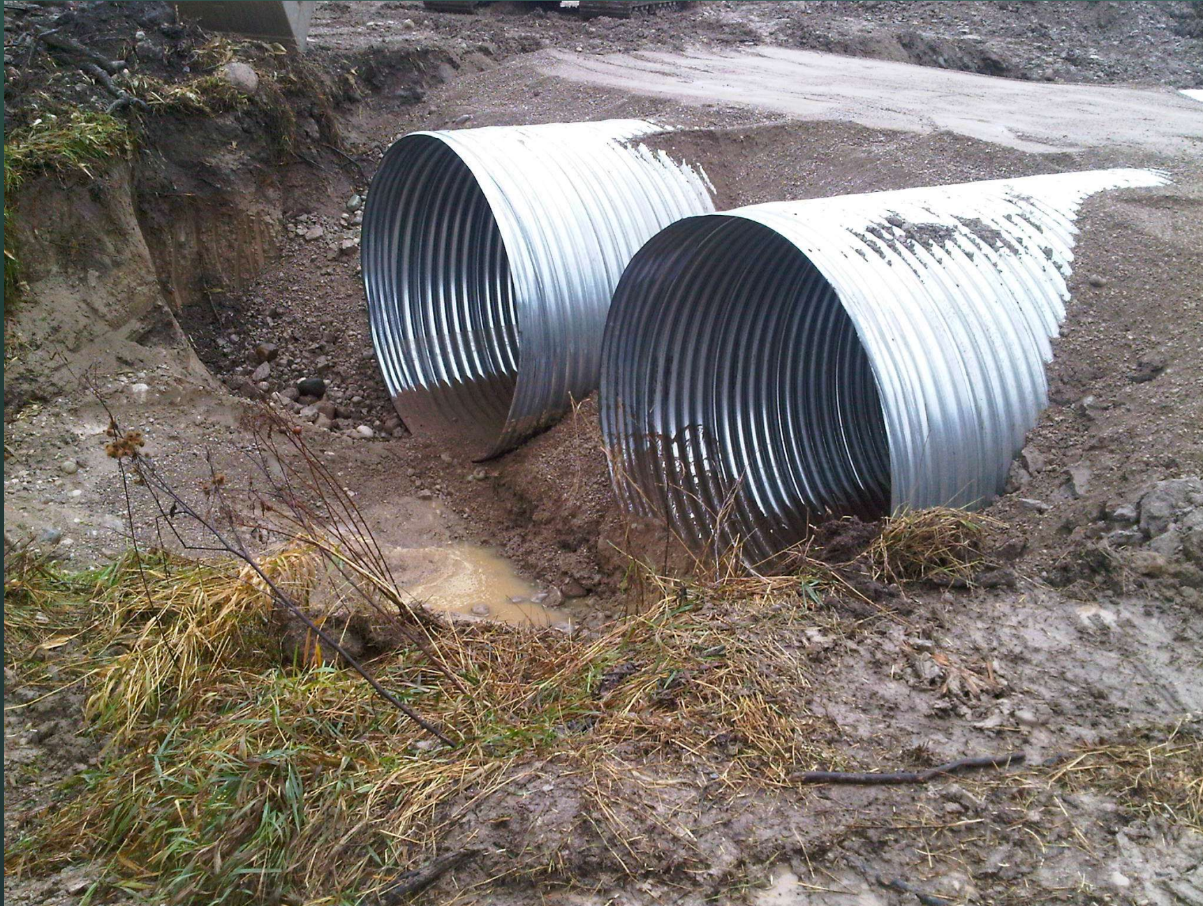
Twin Culvert Installation
