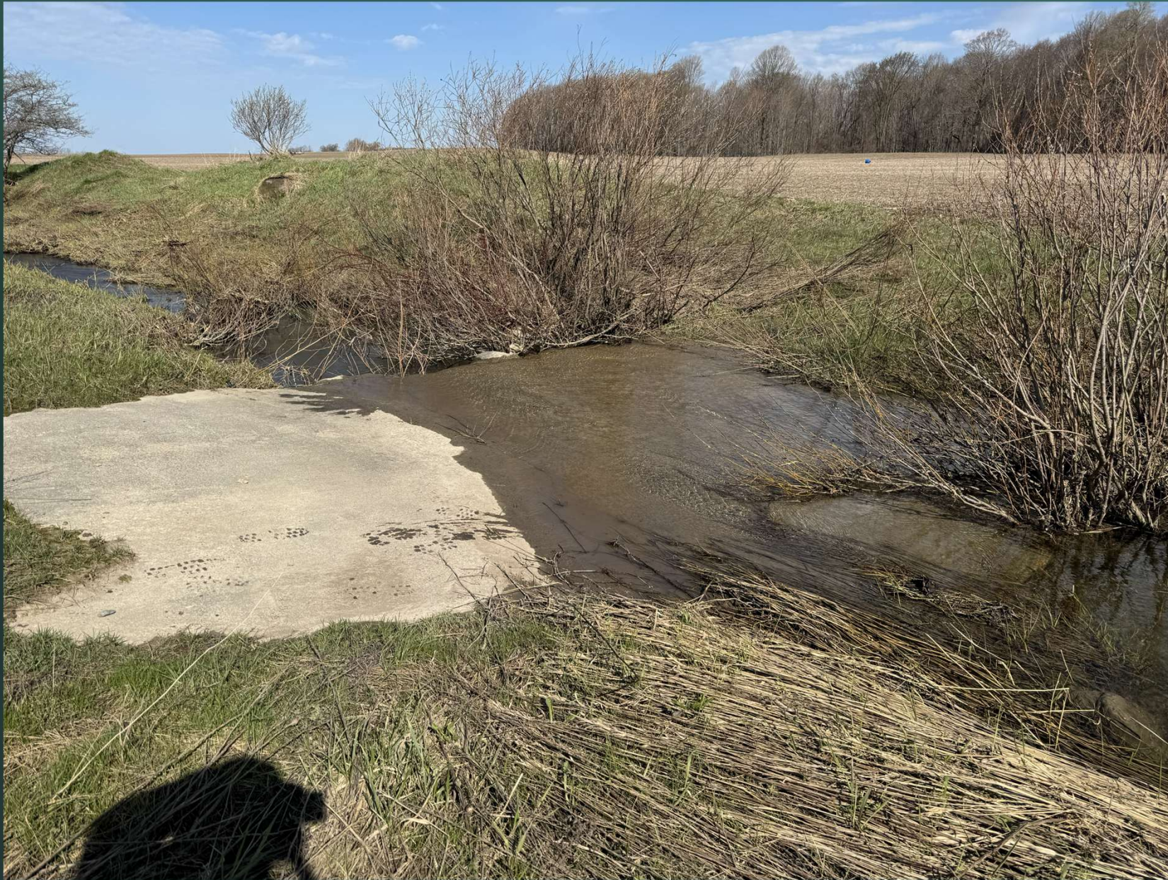
Existing Crossing on Valerie Shortreed Property
