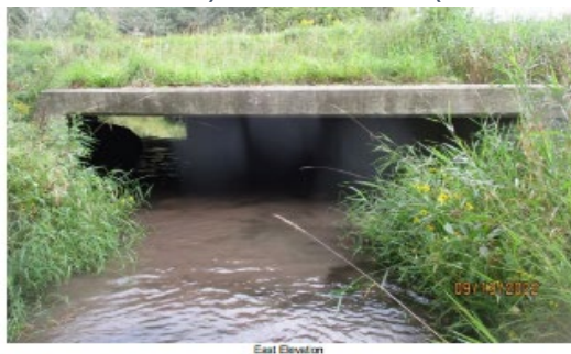
Figure 29 M080 Clyde Line Culvert (BCI=53 Fair)
