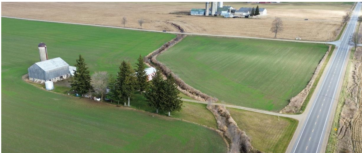
Figure 1 - Facing Northeast, The Bolt Municipal Drain on Lots 5-6, Concession 3 (Nov 2025)
