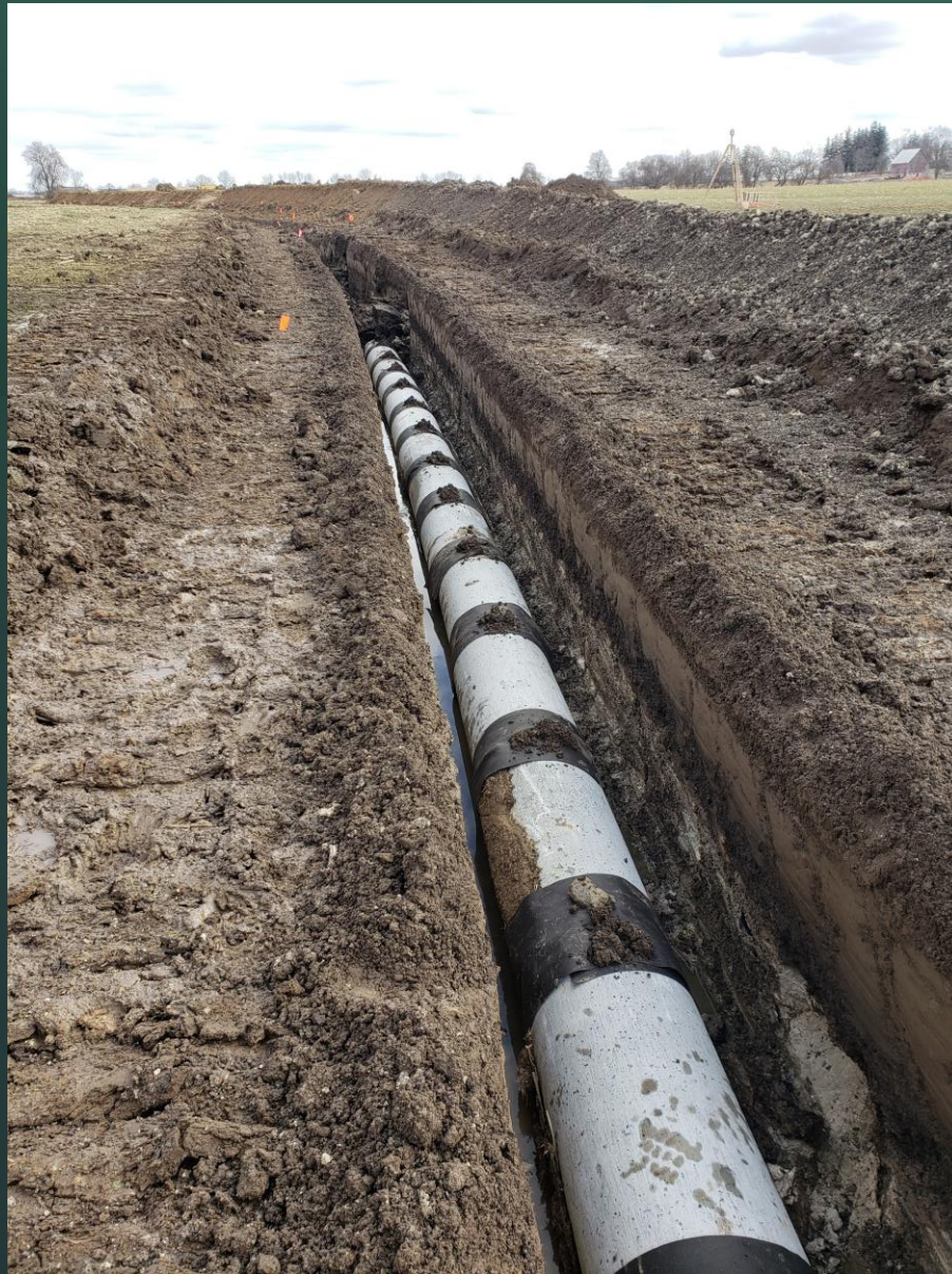
Tile Installation by means of Wheel Machine
