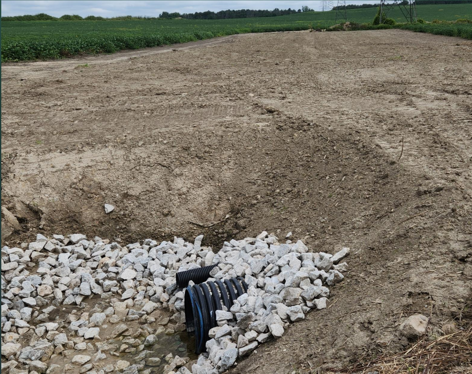
Enclosed Open Ditch
