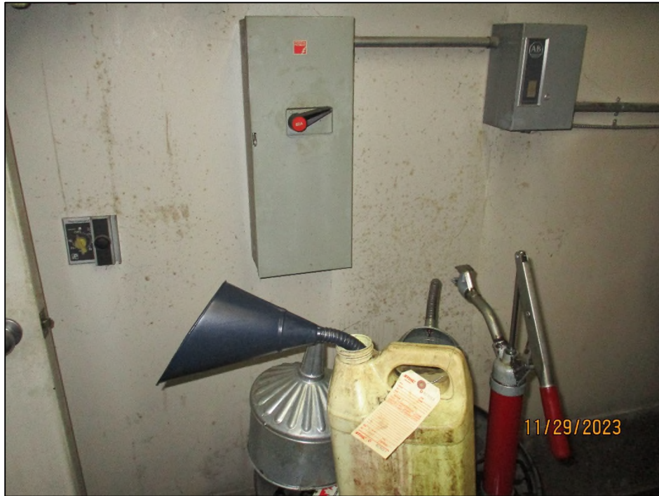
Photograph 3: View of suspect mould spotting on the drywall walls in the Parts Room.
