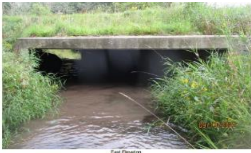
Figure 29 M080 Clyde Line Culvert (BCI=53 Fair)
