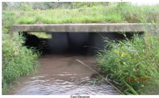
Figure 29 M080 Clyde Line Culvert (BCI=53 Fair)
