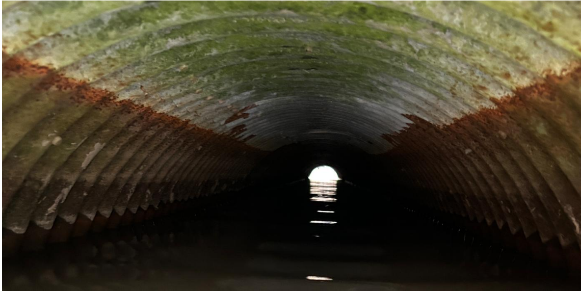
Figure 3 – Inside Bolt Municipal Drain Culvert Crossing of Kieffer Line (Nov 2025)
