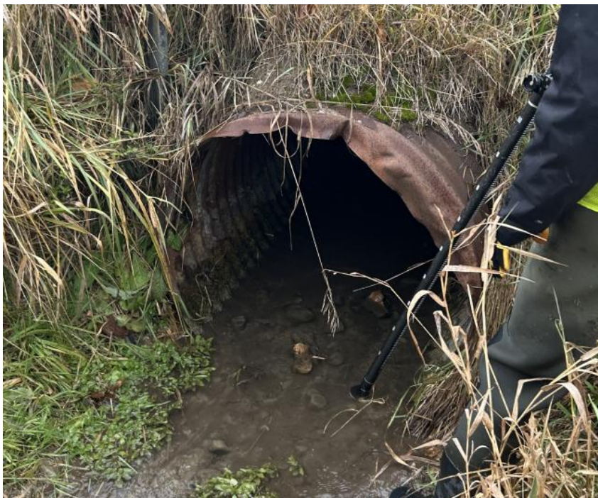
Figure 4 - South End of Bolt Municipal Drain Culvert Crossing of County Road 87 (Nov 2025)
